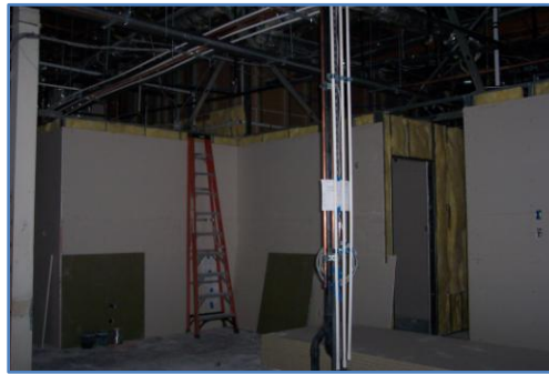
EARLY DAYS: Interior Progressing Nicely
